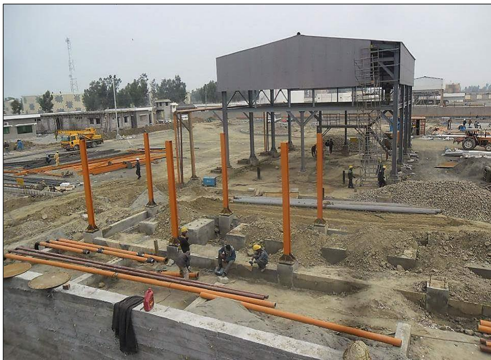
Fig. 4: Construction Works at Site-II.
